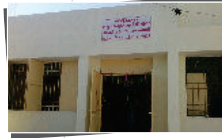
KanyaShala Class Room constructed by REL
